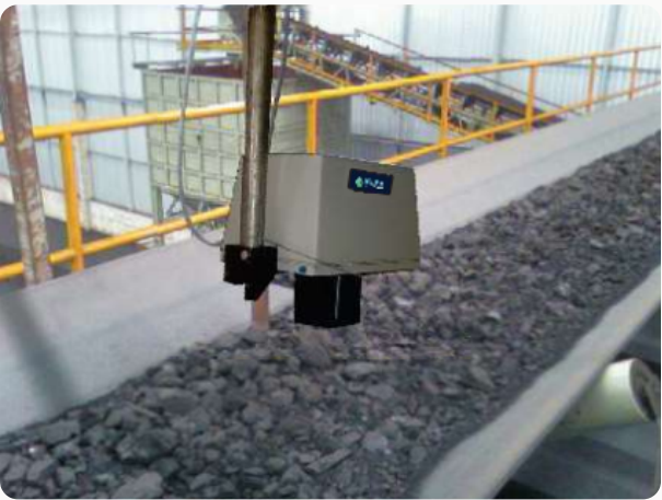
Installation on coke application
